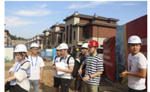
Site visiting of smart construction
