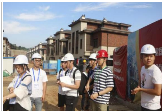
▲ Participants visited the construction site
